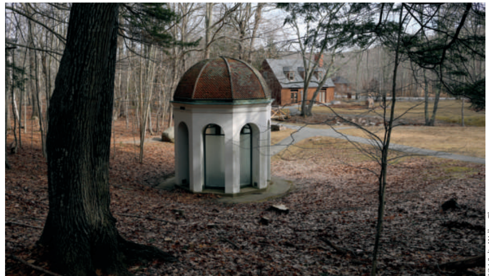
The Sieur de Monts area will have limited access this fall.
