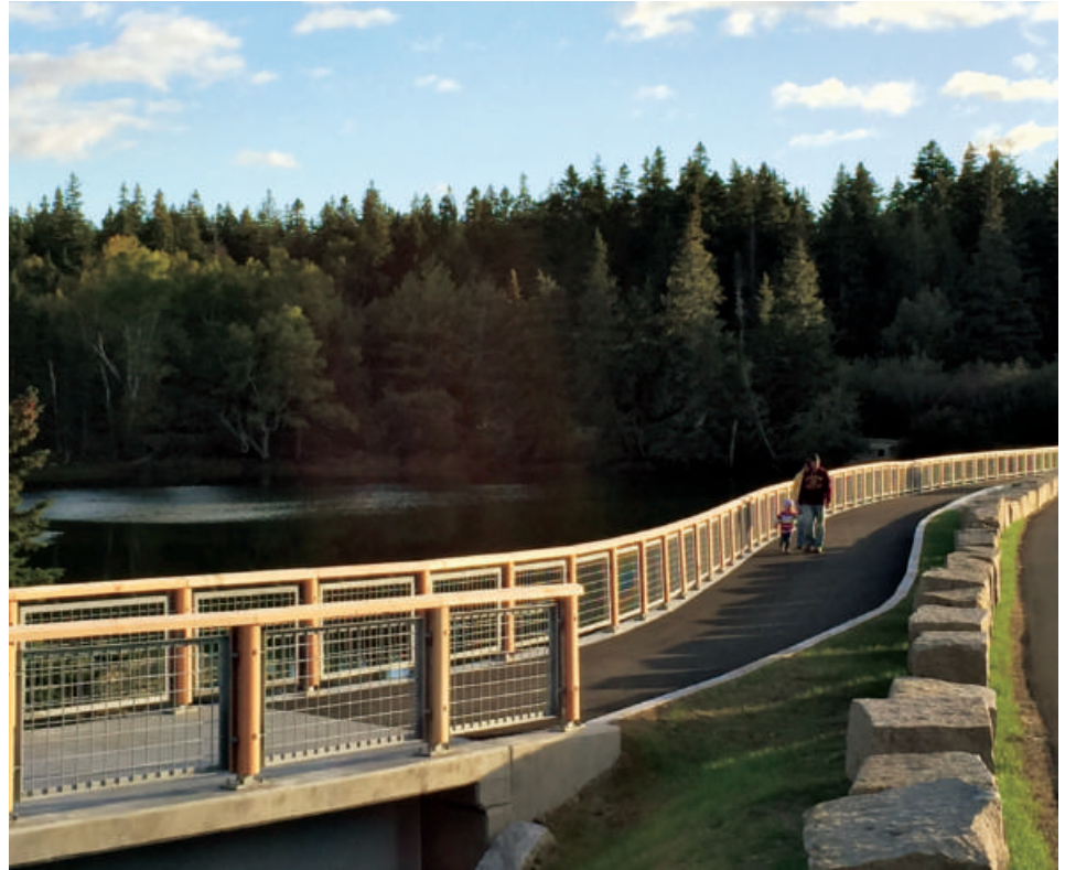
The lovely new bike path alongside the Frazer Creek causeway separates bikers and pedestrians from autos on the causeway, providing a safer crossing for all.
