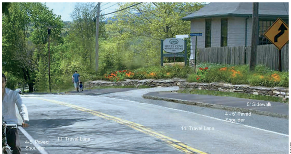
Conceptual illustration of new sidewalk and shoulders on Rte. 3 in Hulls Cove.
