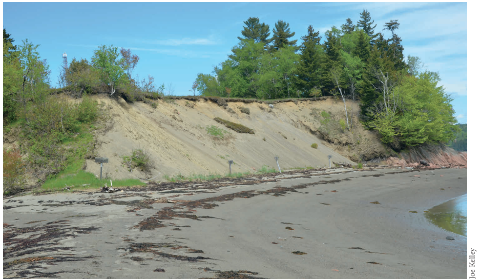
An eroding bluff on St. Croix Island.
