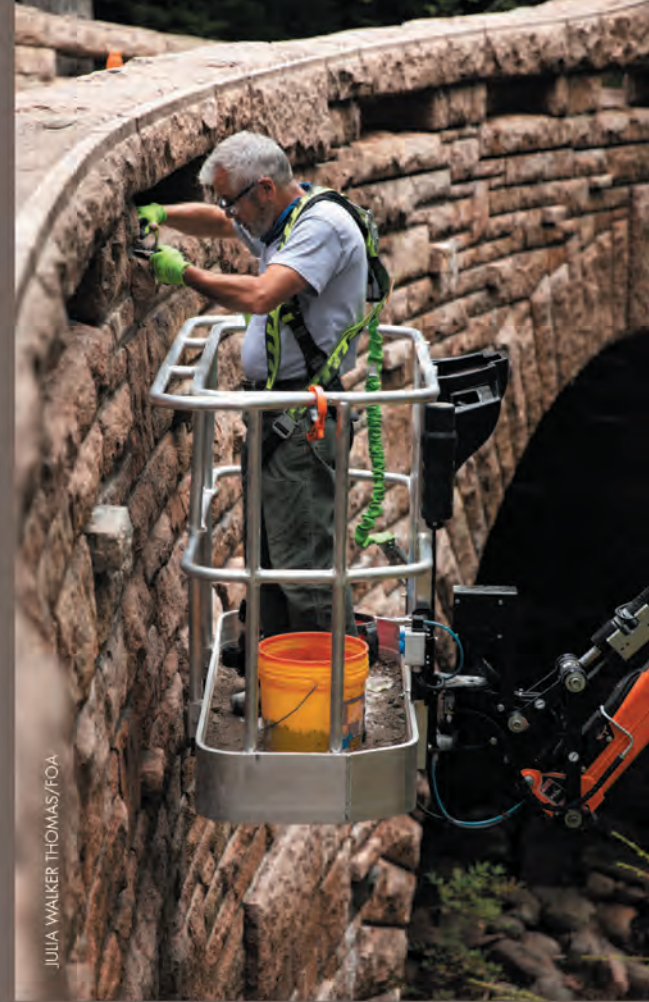
ABOVE: Acadia National Park Master Mason Mike Fitzpatrick replaces mortar on the Amphitheater Bridge.
