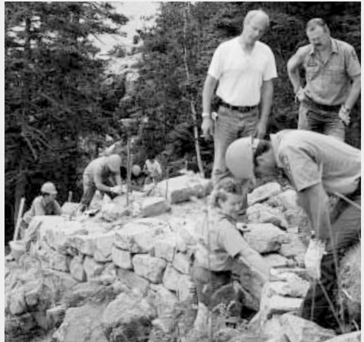
1) Trail crew training on Ocean Path stone retaining wall
