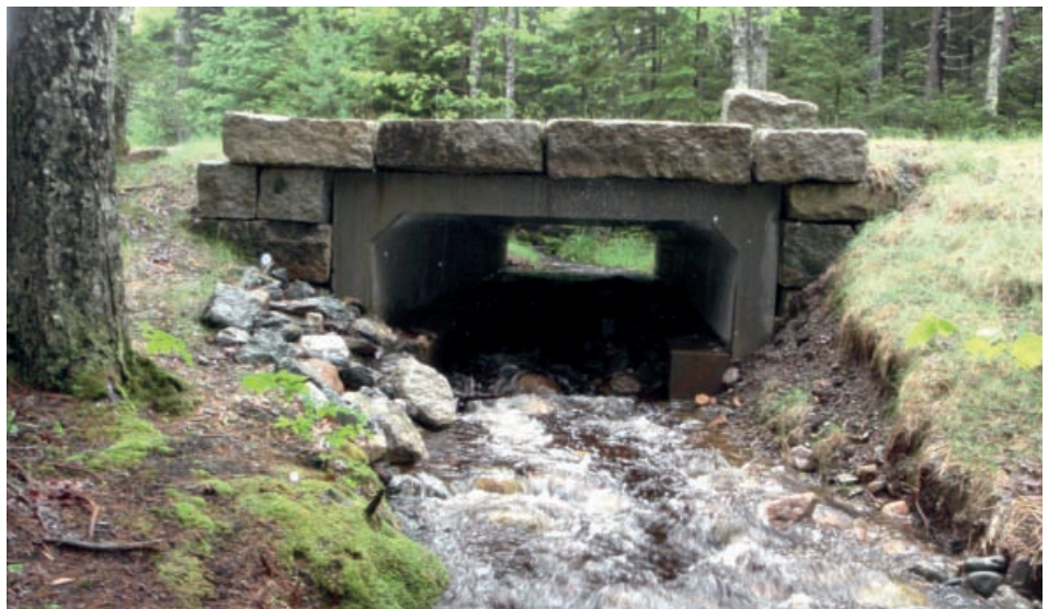
Culvert replacement on the Stanley Brook tributary off Wildwood Stables Road. Before restoration (top), the corrugated metal culvert is perched above the stream and poses a barrier to fish passage. After restoration (bottom), the concrete open-box culvert allows unimpeded fish movement and accommodates greater stormwater flow.
