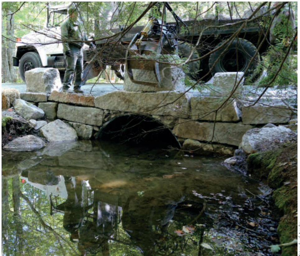
Acadia's roads maintenance crew set new coping stones above the Eagle Lake watershed's new culvert.
