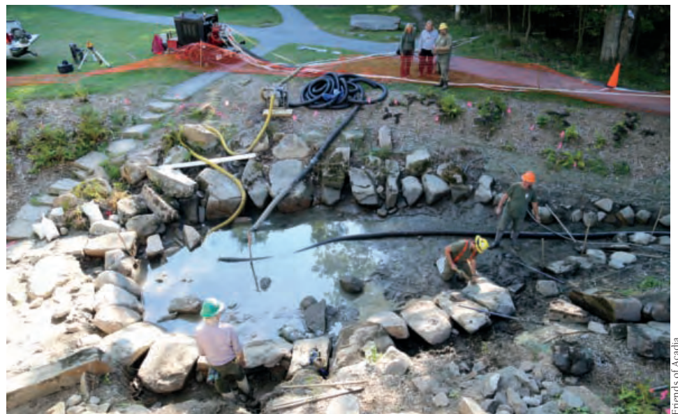
The ANP trails crew reset the historic stones around the pool.
