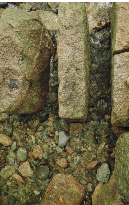
Drainage rock work along Jordan Pond Trail.
