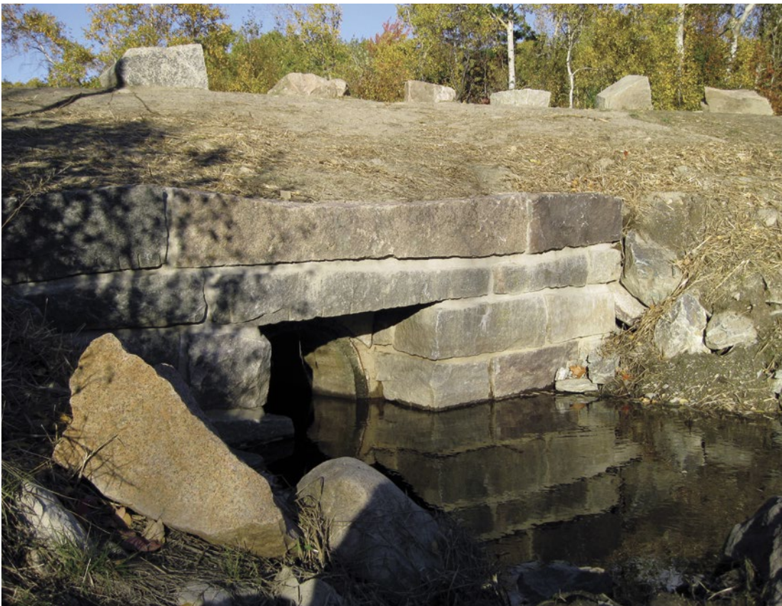
This undersized culvert, located where Cromwell Brook passes under the Park Loop Road, is the sole drainage for the entire Great Meadow wetland. When the Loop Road was constructed in the early decades of the park's existence, it significantly altered the natural hydrology of the area.
