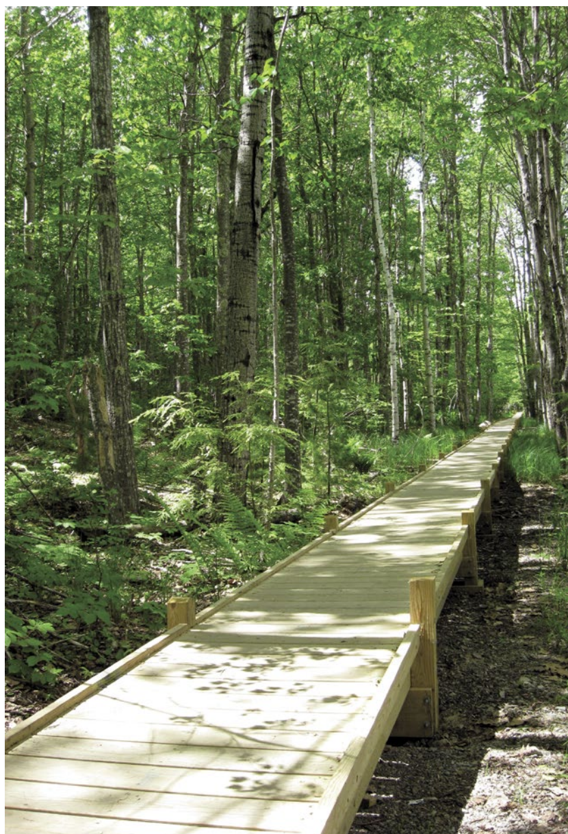
Acadia National Park trail crews and natural resource managers worked together on the 2009 restoration of the historic Jesup Path. The elevated boardwalk allows water to flow freely while keeping hikers high and dry during the wet spring season.
