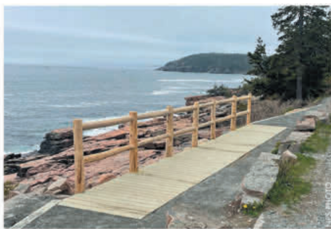
FRIENDS OF ACADIA FUNDED temporary repairs at Ocean Path, including a new bridge and railing where erosion washed away the trail.
